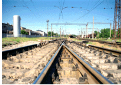
A Main-Line Railroad Switch
