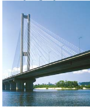
Pivdenny bridge, Kyiv
